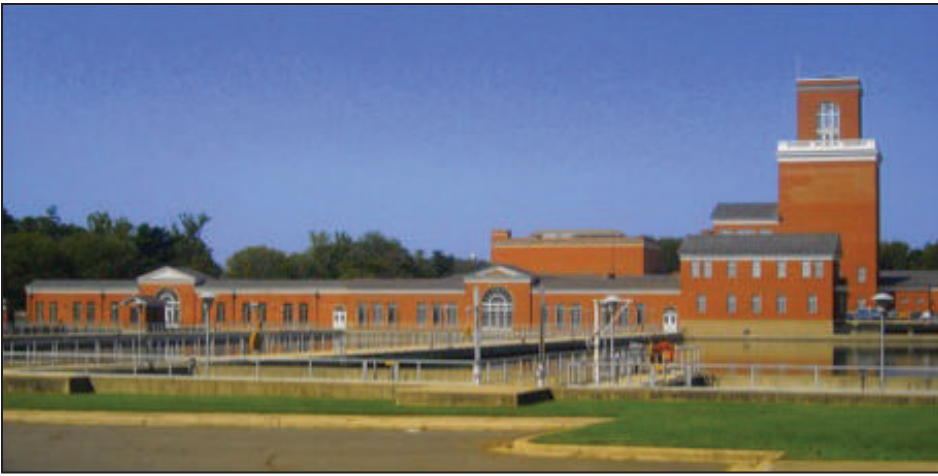
Left: Dalecarlia Water Treatment Plant, Washington, DC By AgnosticPreachersKid - Own work, CC BY-SA 3.0, https://commons.wikimedia.org/w/index.php?curid=6026048
